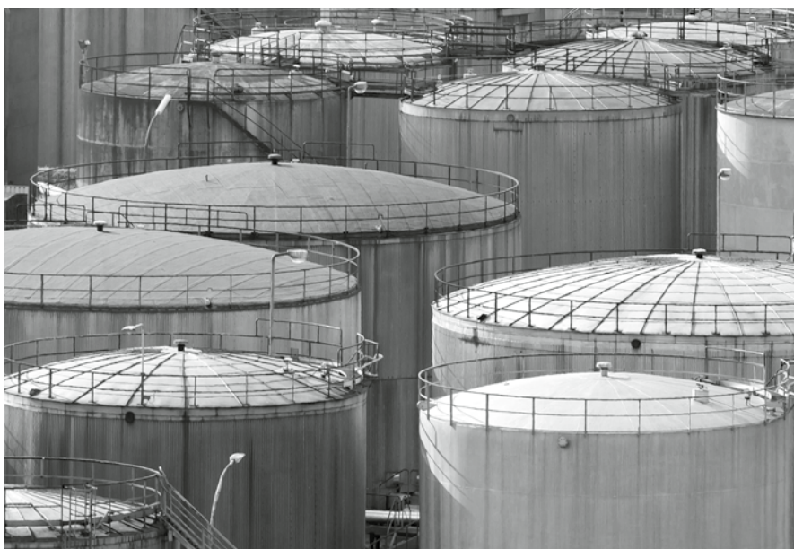
HAMBURG By-products and end products are stored in the on-site tank farm.
